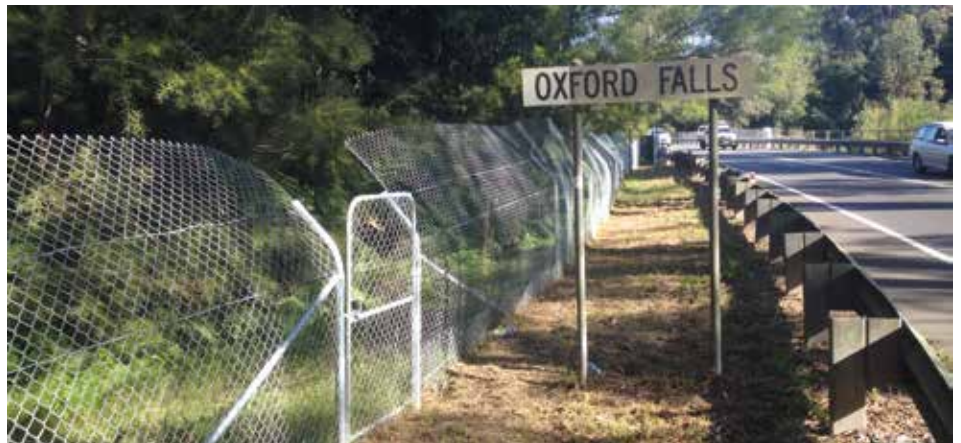
The 98 metre fauna fence installed along the Wakehurst Parkway.
